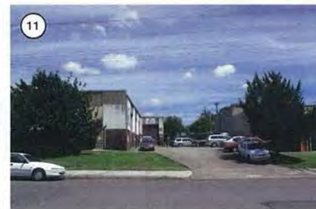
Existing industrial buildings along Shepherd Street
