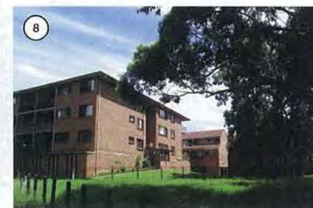
Residential apartment buildings to the north of Atkinson Street
