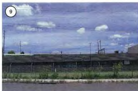
Existing industrial buildings along Shepherd Street
