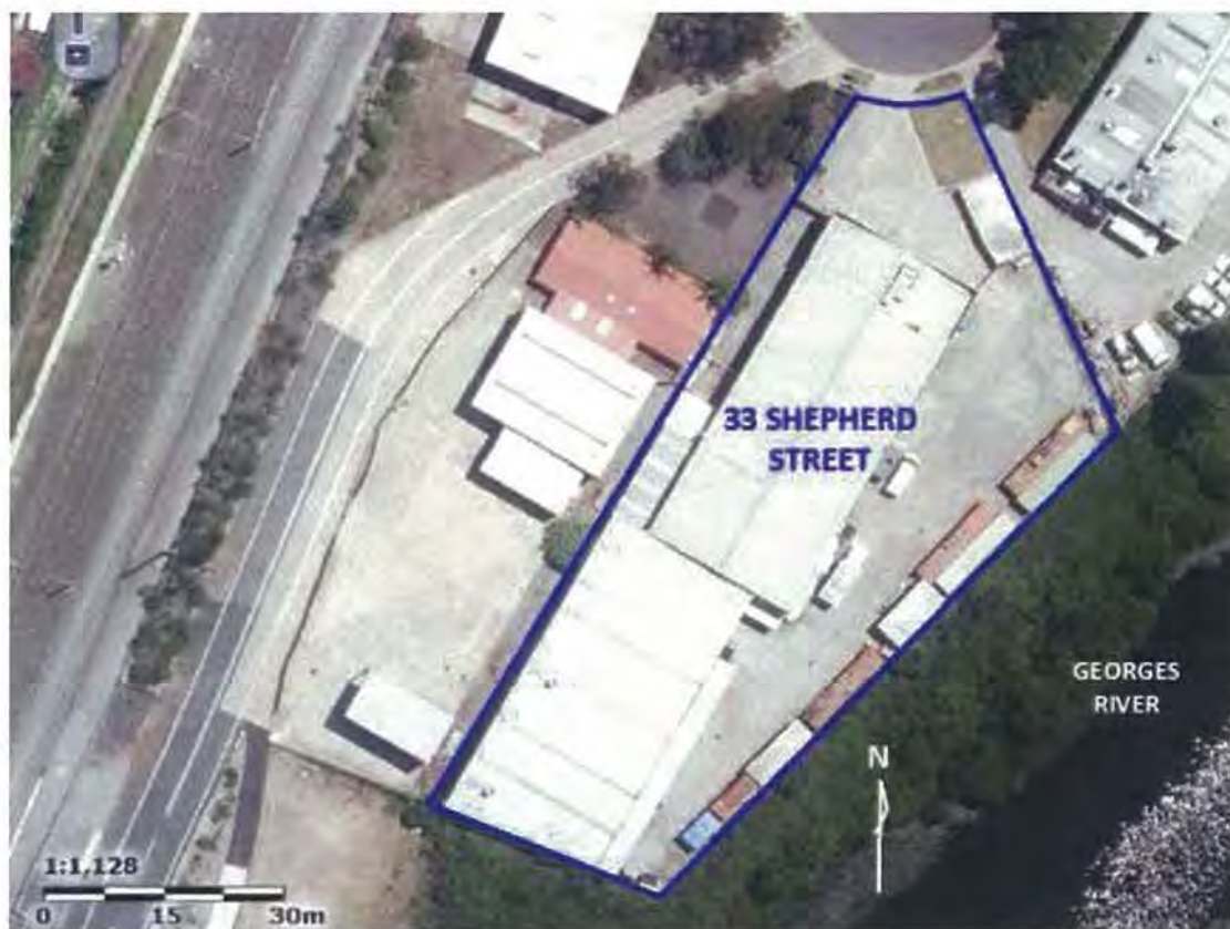
Figure 13 - Site location at 33 Shepherd Street, Liverpool, an operational factory establishment with no vegetation occurring within the site except for a small patch of Kikuyu. The eastern boundary of the site demarcating vegetation along a section of the western embankment of the Georges River.
